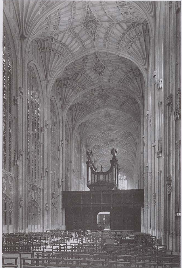
The chapel of King's College, Cambridge, with its fan-vaulted roof and large areas of glass and delicate stone work, marks the highest point of Gothic architecture in England. The vault was completed at the beginning of the sixteenth century, and the wooden organ screen across the centre of the chapel is of Tudor design.
