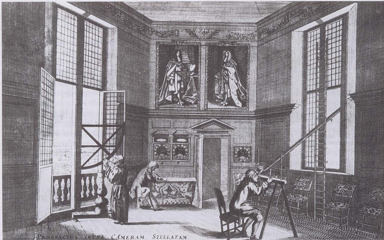
The Royal Observatory at Greenwich was founded by Charles II, who had a great interest in scientific matters. On the left a quadrant is being used, larger but similar to those used for navigation on ocean-going ships. On the right an extremely long telescope is being used to observe the heavenly bodies.
